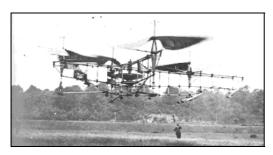
In 1920, Etienne Oemichen, an employee of the French Peugeot car company, built a quad-rotor machine in a similar style to that of de Bothezat, but with eight additional rotors for control and propulsion. His machine typified the cumbrous mechanical complexity of the helicopters of that time. His initial design was under-powered, and it had to have a hydrogen
