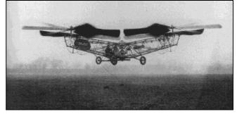
de Bothezat (1919). De Bothezat's machine was a quadrotor with a rotor located at each end of a truss structure of intersecting beams, placed in the shape of a cross. Ivan Jerome was the codesigner. Each rotor had six wide chord blades. Control of
