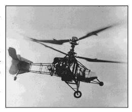
hinges. The blades were controlled in cyclic pitch using a swashplate design. Yaw control was achieved by differential torque on one rotor with respect to the other rotor. Horizontal and vertical tails were used for increased stability. For its time, the aircraft had held several FAI records, including a duration flight of 62 minutes and distance flown of 44 km (27 mi). Further work on the Breguet-Dorand machine was stopped prior to the outbreak of World War 2.
