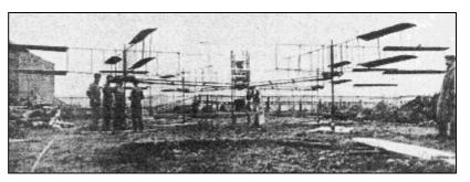
a few seconds at low altitude, but this has never been satisfactorily verified. Certainly, the 24-hp engine used in the machine was hardly powerful enough to have sustained hovering flight out of ground effect.
